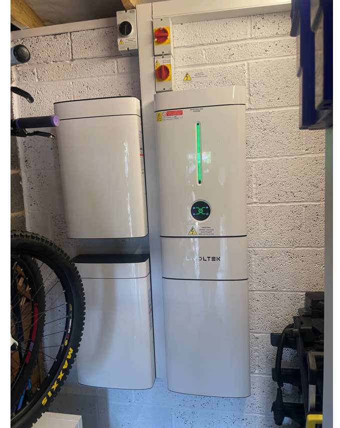
All in One 5kW inverter/15 kWh battery
