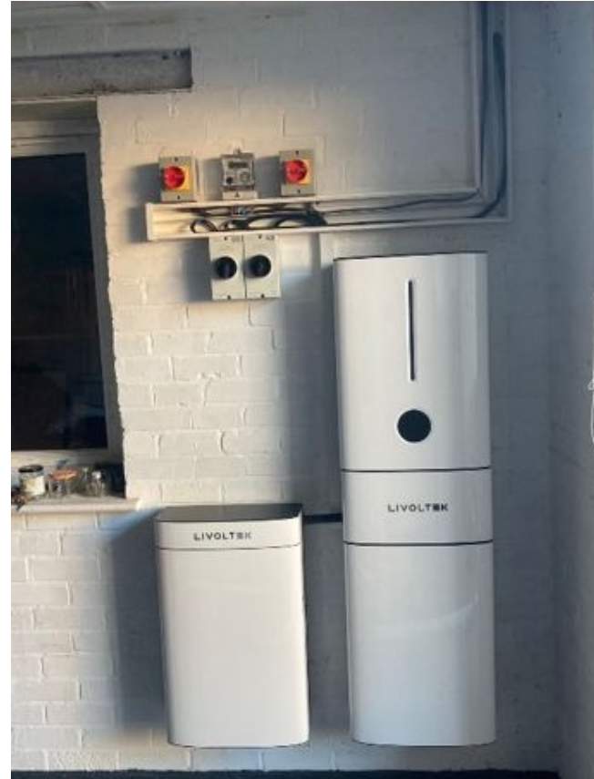
All in One 5kW inverter/10 kWh battery
