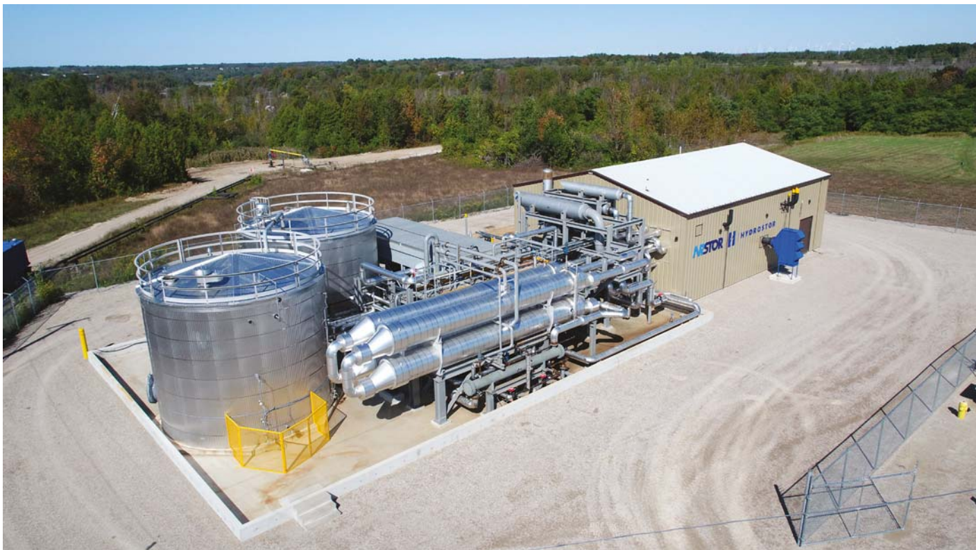
NRSTor and technology provider Hydrostor completed the world's first advanced compressed air energy storage plant (pictured) in 2019.
