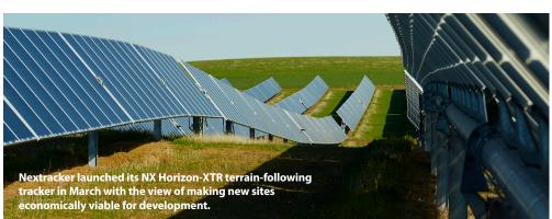
"Deploying traditional trackers on sites with varied terrain has required extra earthwork and longer foundation piles, which increases project costs and adds risk. Earthwork is especially painful as it affects a solar project three times: first performing grading, next reseeding the exposed dirt and later fixing the inevitable erosion and hydrology issues that come from the lack of well-vegetated topsoil."
