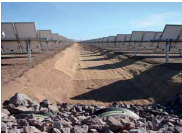
Design for high water flow diversion. Do not assume large, sudden storm events can pass over a facility without water depth and velocity damage. Consider conveying large flows around the site rather than flow over land
