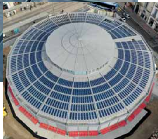
Roof of newly constructed old style "Art Nouveau" market place in the historical center of Montpellier city ; 900 double glass with biomimetic cells designed by S'Tile.
