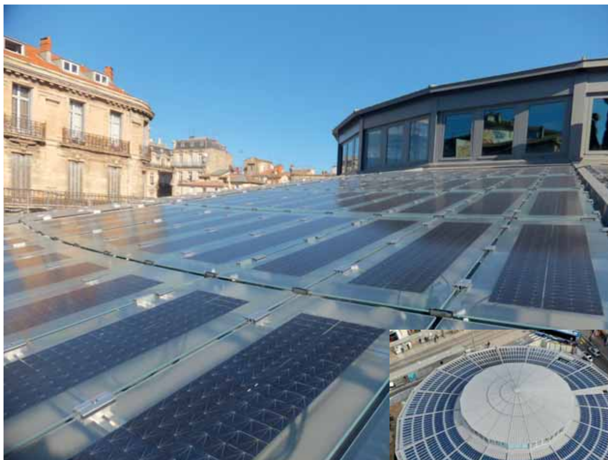
Roof of newly constructed old style "Art Nouveau" market place in the historical center of Montpellier city ; 900 double glass with biomimetic cells designed by S'Tile.
