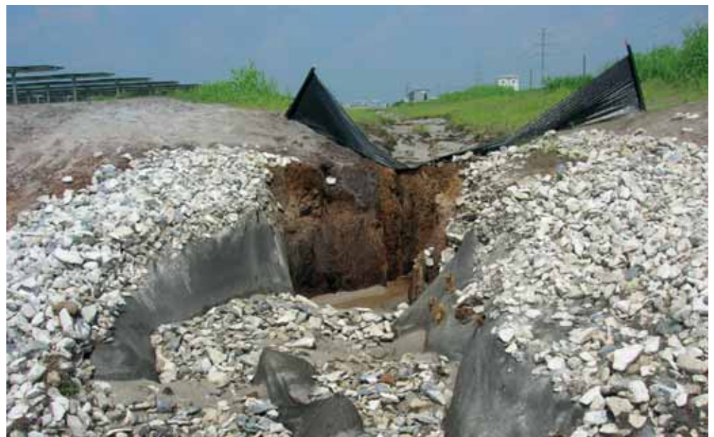
Proper installation of erosion control materials is critical for function during and after construction of PV power plant, particularly in regions with high rainfall
